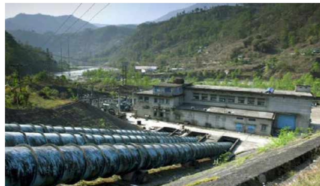
Water Diversion pipes for hydro-power plant on Bhote-Koshi (Photo: Vijay Paranjpye, Field Trip, November, 2019)
