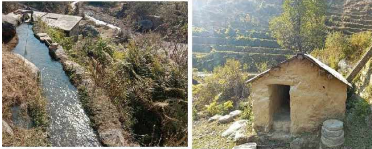
Stream Flow Being Diverted Through A Channel And Water Traveling Down A Wooden Channel Generating Hydraulic Energy, Which Turns The Blades Around A Fulcrum, Which Eventually Turns The Stone Milling Wheels
