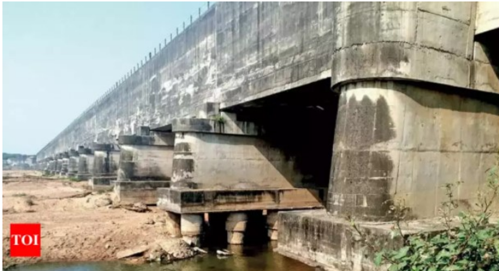
Figure 19: Damages caused to the aqueduct of the Narmada main canal due to erosion
