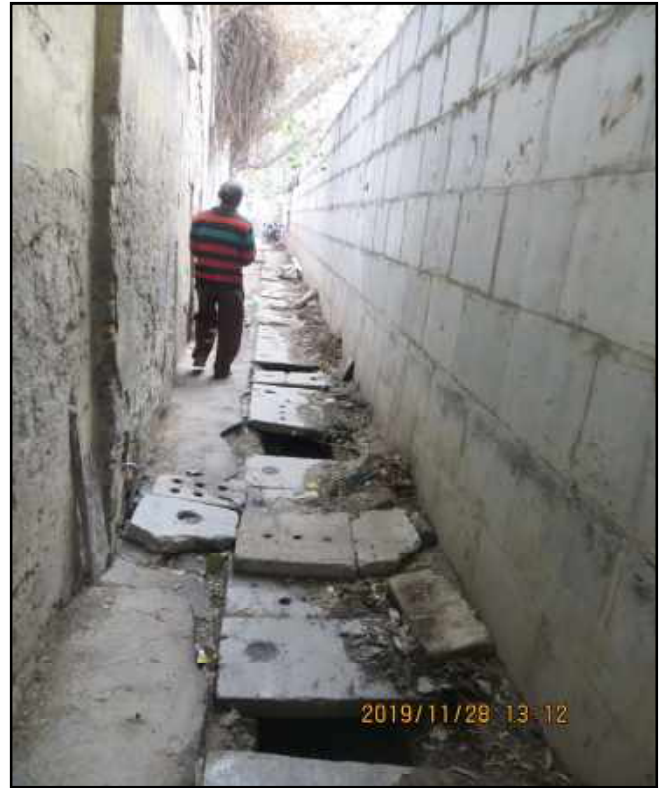
B. Condition of Waste water drain at Yamuna Ghat
