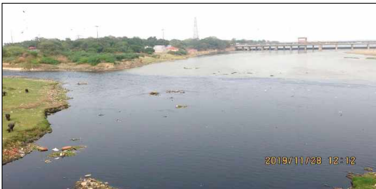
Figure 5: Picture showing discharge of Najafgarh drain in the River Yamuna near Wazirabad Barrage
