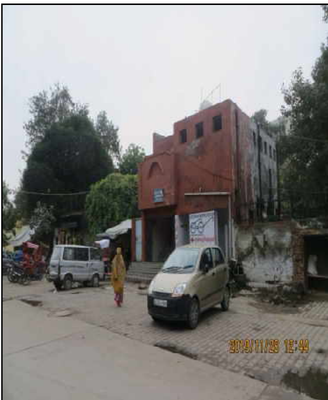
C. Community toilet at Yamuna ghat
