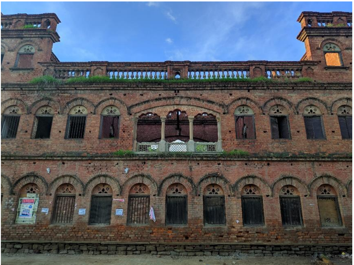
Abandoned Colonial Warehouse on the River, Mirzapur
