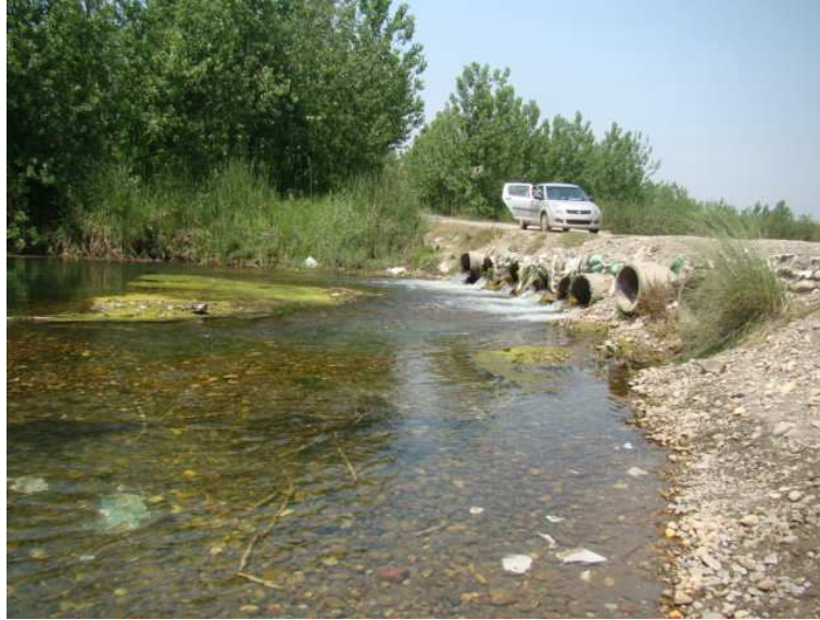
Culvert on river Thapana
