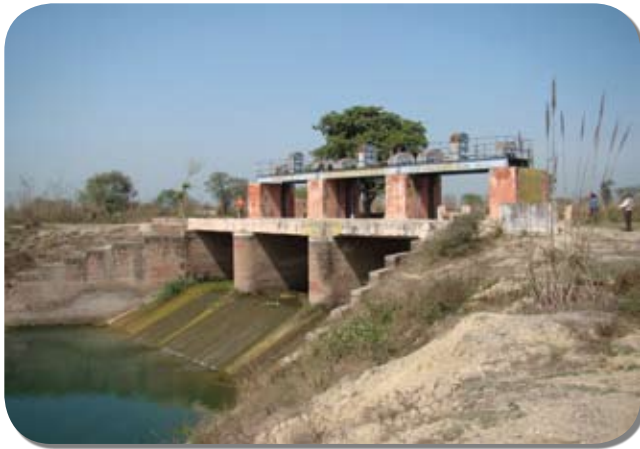
Pic 17: Munak Escape (Drain No 2) at its origin (WYC). 11.3.10
