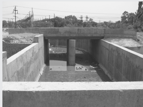
Munak canal (CLC) still under construction!
