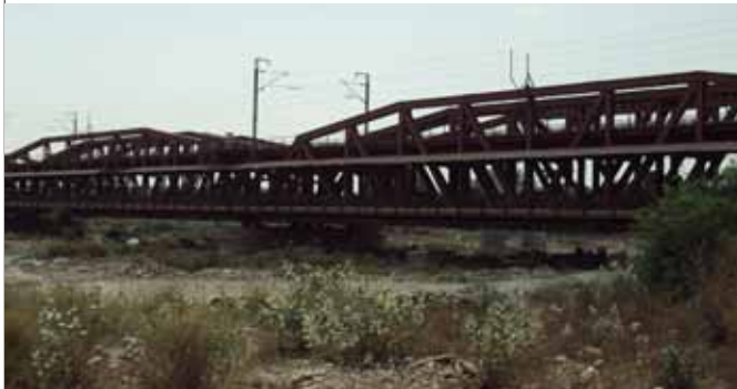
Old Railway Bridge
