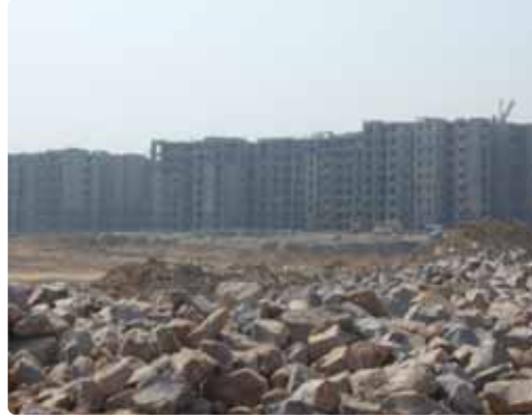
High end apartments being constructed in the games village.
