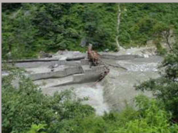
Image 7 : Partially Constructed HEP Head
