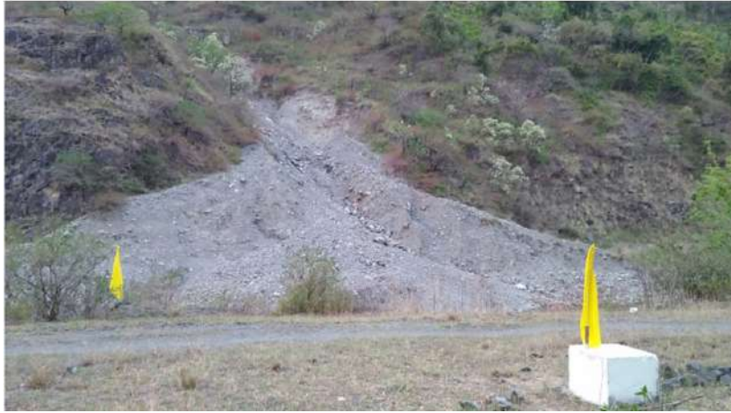
Image 29 : A large Landslide at the Proposed Lakhwar Dam Site
